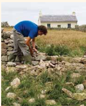
Repairing a dry stone wall near Stoneycroft, Lundy
