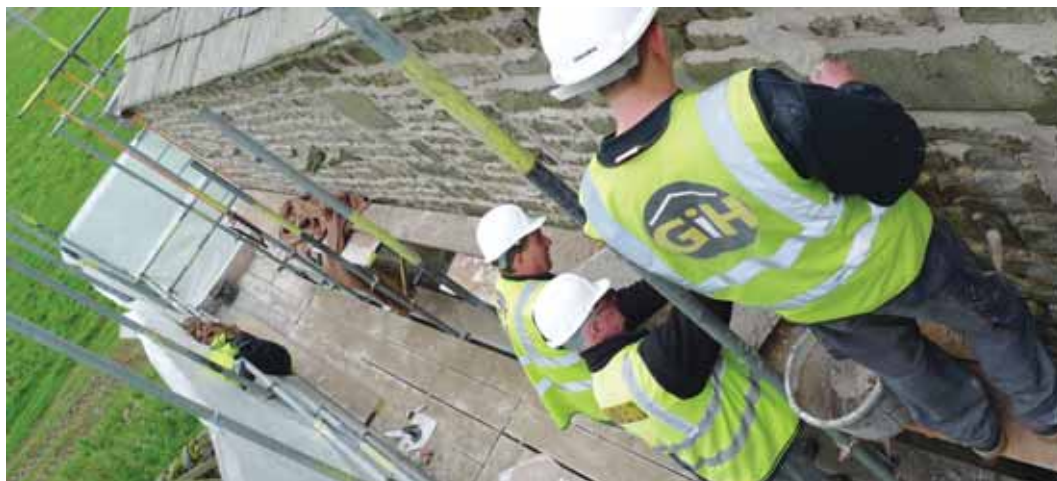
G.I. Hopley contractors repointing Cowside
